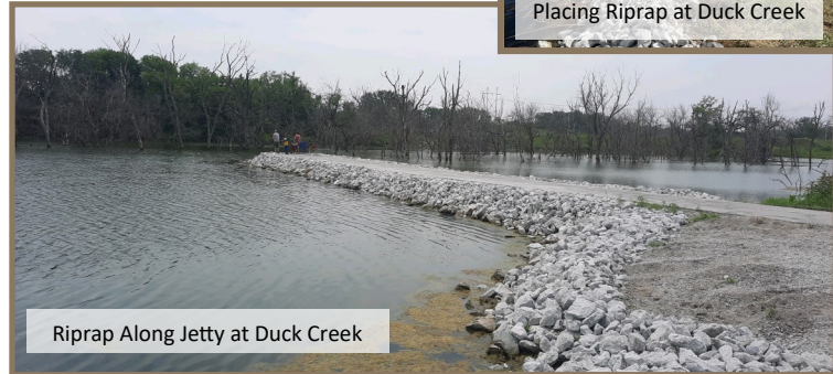
Placing Riprap at Duck Creek
