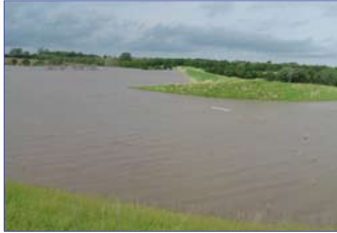
This dam in the Upper Little Nemaha Watershed near Bennet filled to capacity then routed excess water around its spillway following heavy June rains.
