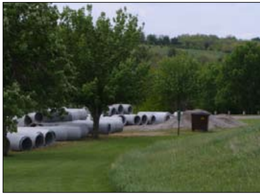
Concrete pipe for renovation project stockpiled near RV camping area at Iron Horse Trail Lake
