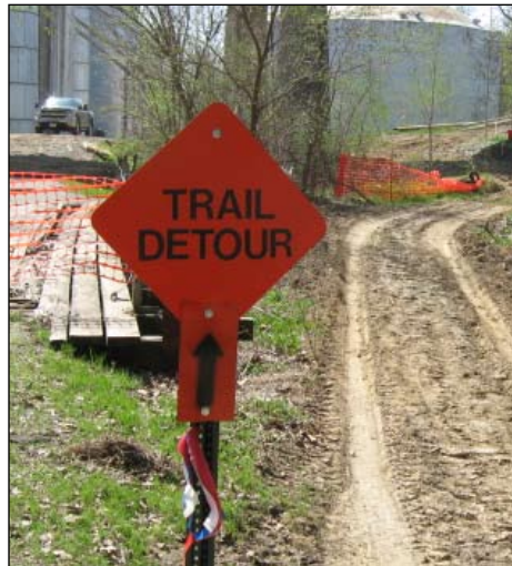
Trail detour around Missouri River bridge construction at Brownville.
