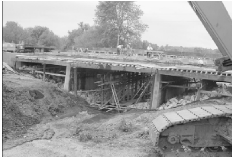
Construction progresses on the bridge across Weldon Creek.
