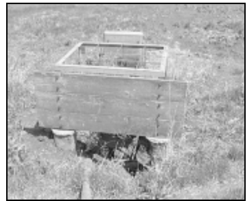
Brownell structure 13-6 riser before repair work
