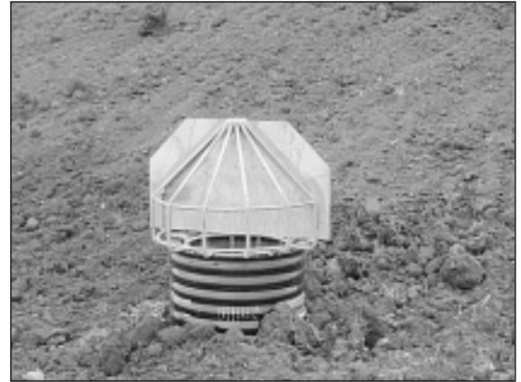
Brownell structure 13-6 riser after repair work
