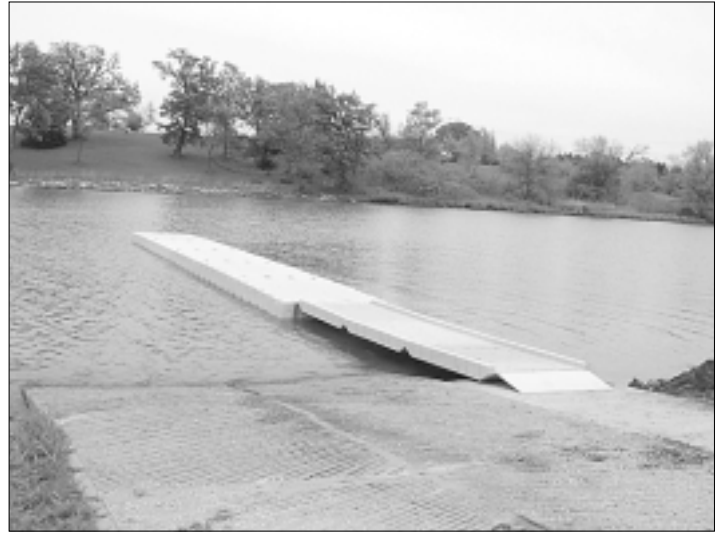
This new dock is now in place at Kirkman's Cove.
