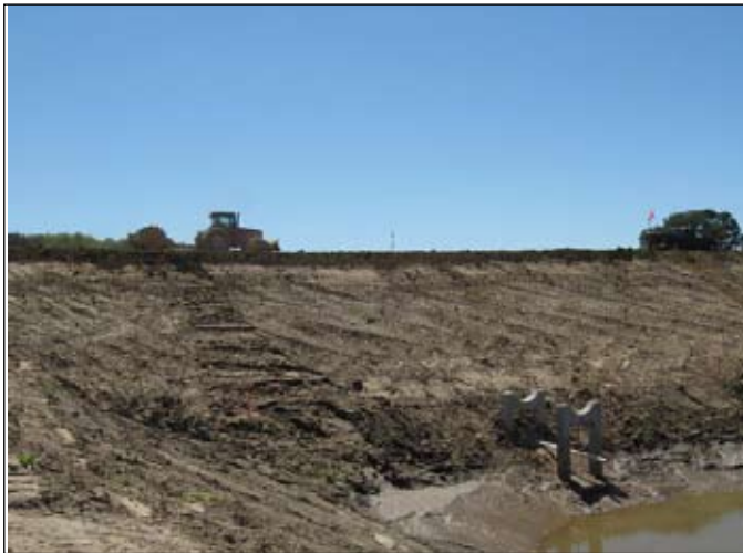
“Work continues on the Buck Creek dam near Peru.”
