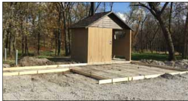
The contractor prepares to pour concrete for restrooms at Duck Creek Recreation Area.
