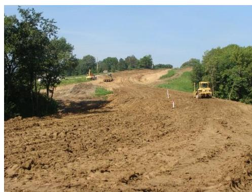
← Kreifels Conservation is doing the earthwork phase for relocation of the county road, which would have been inundated by water from the lake project. Once dirt work is done and has time to properly settle, the next step is to install a bridge and a box culvert. This road project will result in replacement of two aging bridges and provide a safer road that will allow for heavier vehicles and less maintenance.
