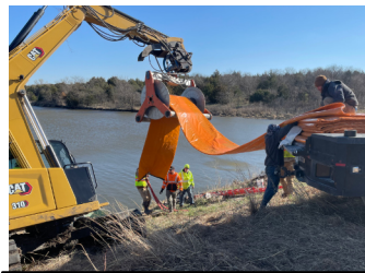
Above: Workers install a UV-CIPP liner into an outlet pipe.
