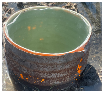
Above: A Vertical outlet pipe after rehabilitation, the original corrugated metal pipe corroded and developed holes over time. An orange UV-CIPP liner forms a durable new pipe inside the existing structure.
