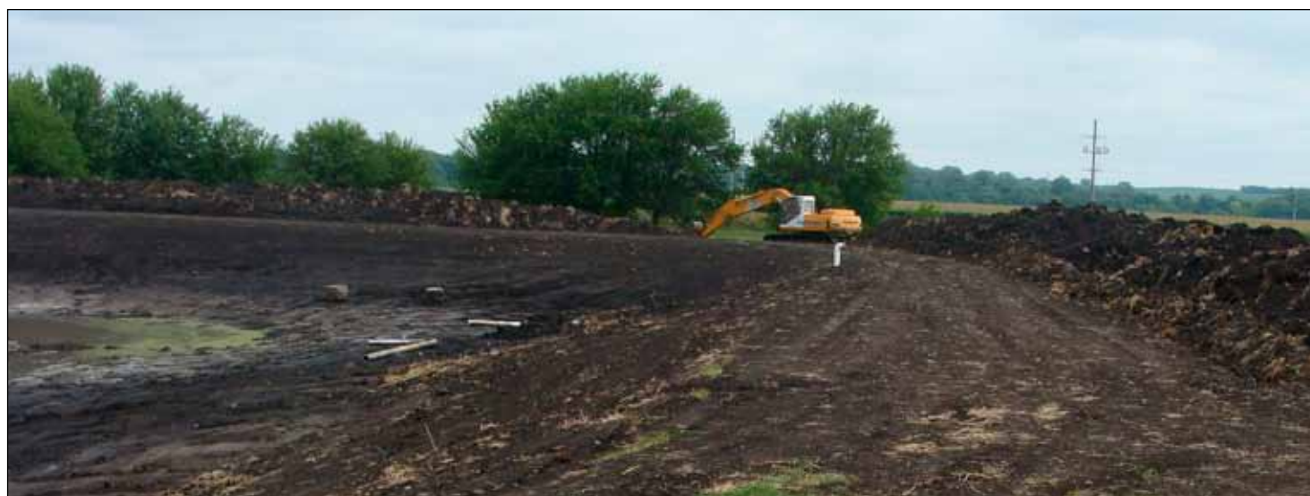
Right: Sediment removal was a large part of the project to improve Gritzka Lake in Talmage last year.
