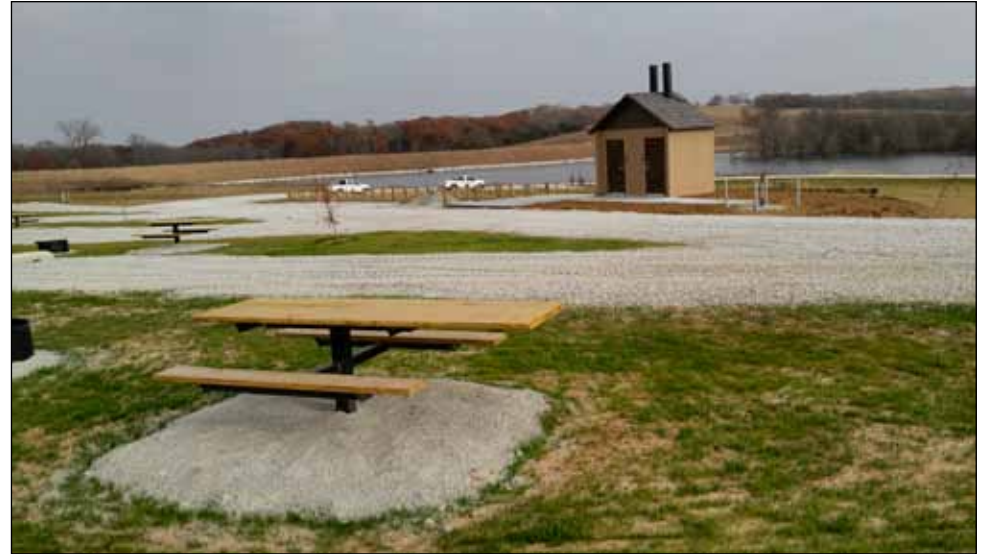
Restrooms, concrete, picnic tables and water are ready to go at Duck Creek Recreation Area.
