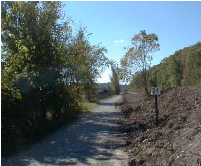
Drainage work and sections of paving are planned for this area of the Steamboat Trace.
