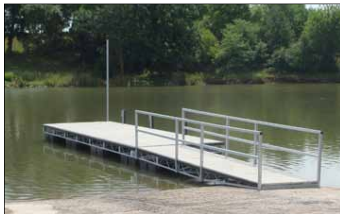
The new dock at Kirkman's Cove installed in July, 2016
