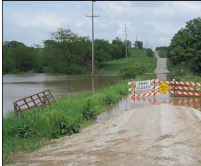
Once completed the water across the road in this photo will flow through the box culvert under the road instead.
