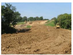
← Kreifels Conservation is doing the earthwork phase for relocation of the county road, which would have been inundated by water from the lake project. Once dirt work is
